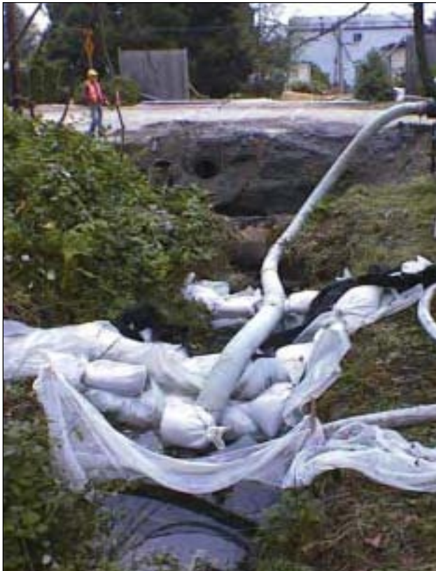
A stream bypass used to divert water around a construction site
