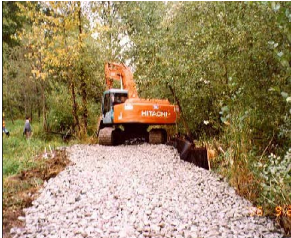
Access road installation
