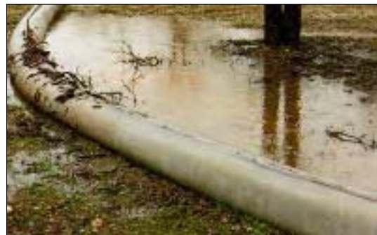
Continuous berm intercepting water from construction area
