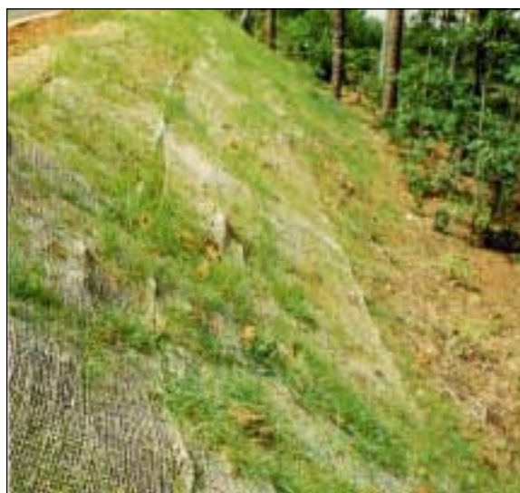
Stabilizing the soil using matting and hydroseeding
