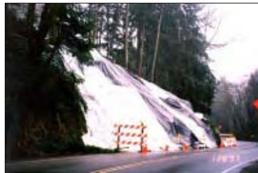
Plastic covering used as a temporary erosion control on slope at slide area after storm and before repair
