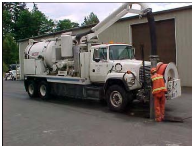
Vactor truck removing sediment from catch basin
