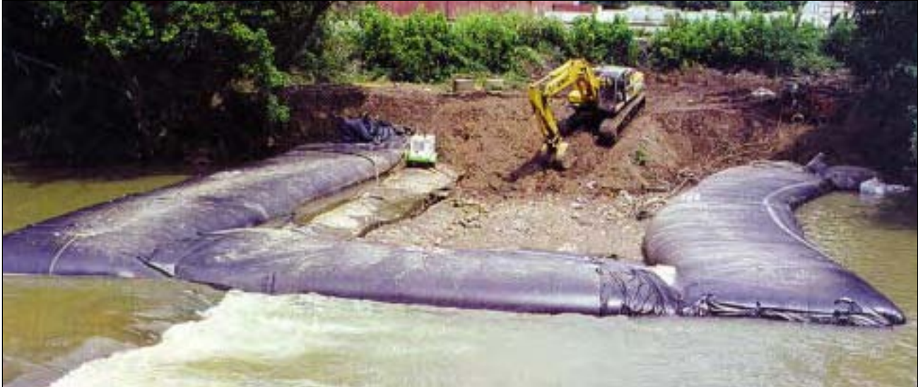
Aqua barrier used as coffer dam
