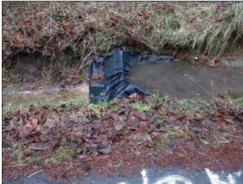
A triangular silt dike in place with accumulated sediment being retained on site, prior to cleaning
