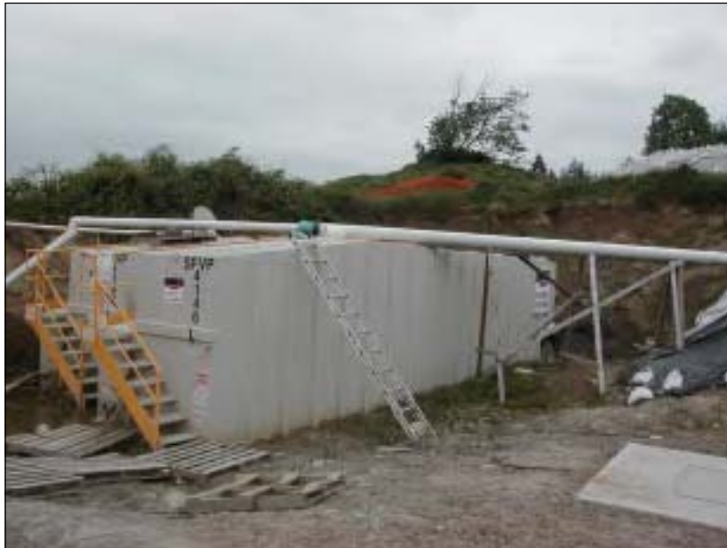
A settling tank in use to allow onsite containment of water borne soil particles
