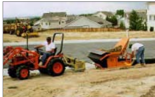
Continuous berm retaining soil particles and debris
