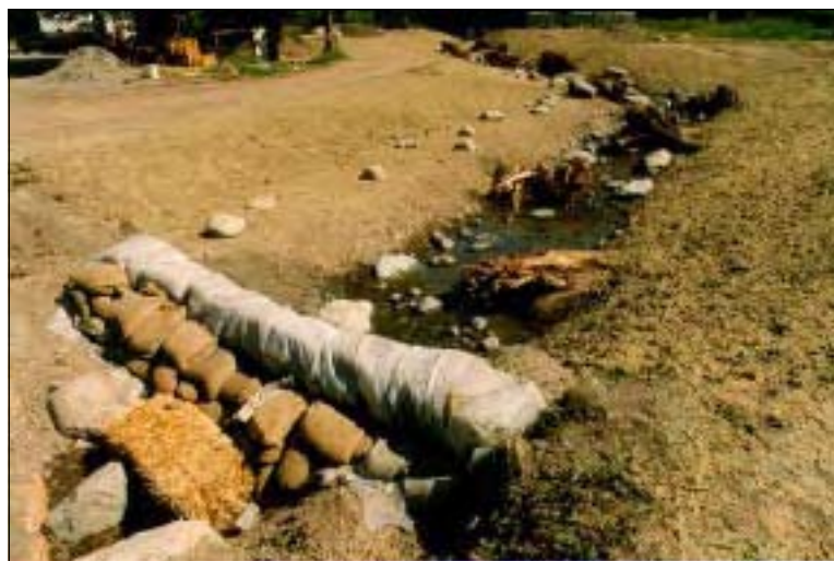
Sandbags used in combination with plastic and strawbales serving as a barrier
