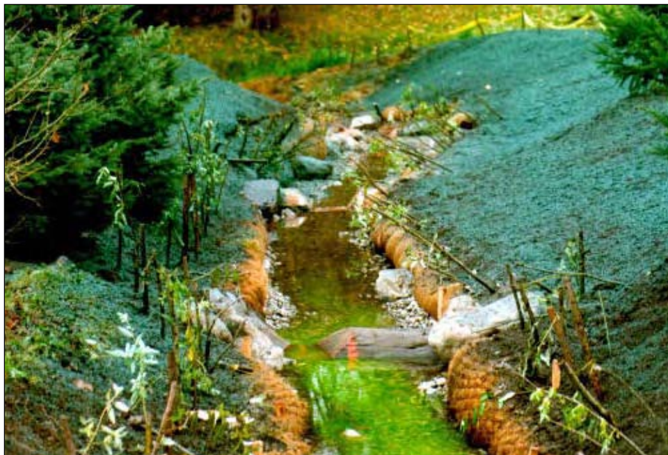
Stabilizing the stream bank by using coir logs, hydroseeding, and live staking. Streambed gravel installed to provide a natural spawning substrate
