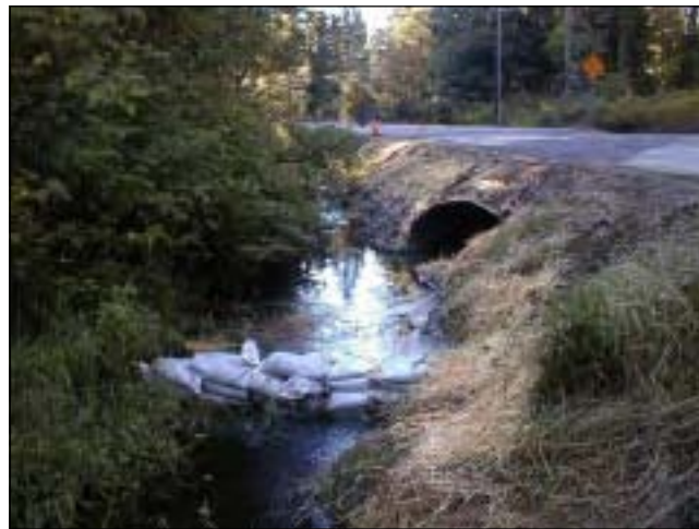
Sandbags acting as a barrier
