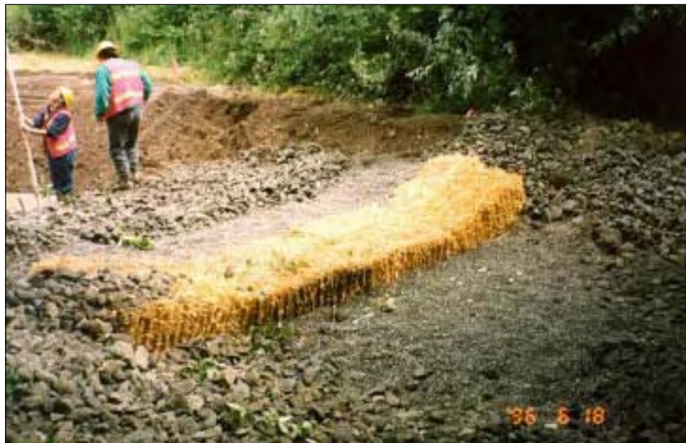
Straw Bale Barrier (3) being used with a rock spillway decreasing runoff velocity and retaining sediment onsite
