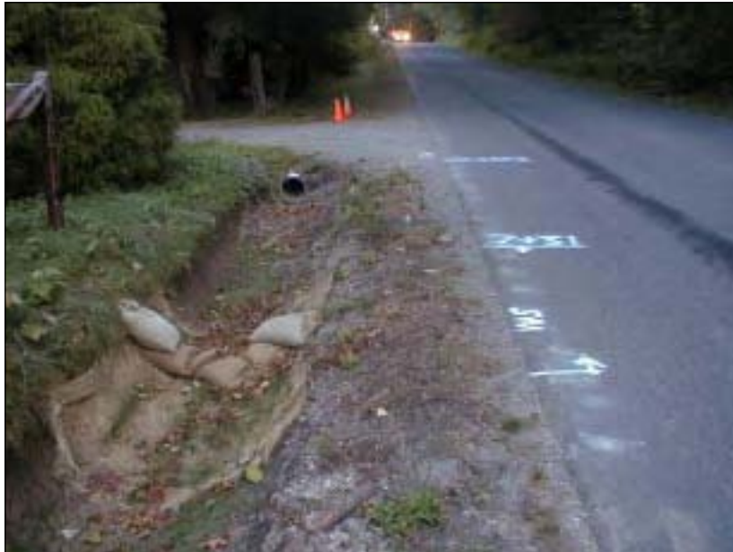
A sandbag barrier used to decrease water velocity. Note use of silt mat and hydroseeding to decrease erosion and to increase vegetation in channel
