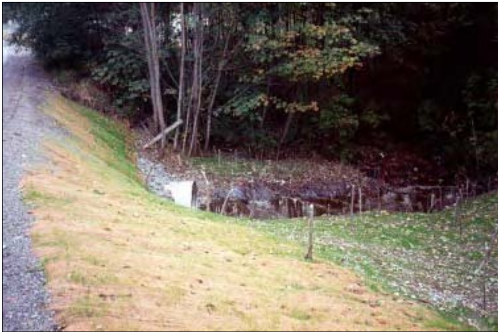
Using straw and live staking to reduce erosion and provide vegetative cover once vegetation has established
