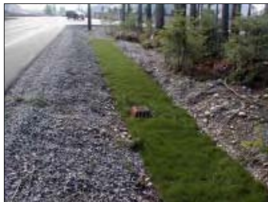
Grass lined channel: providing a filter
