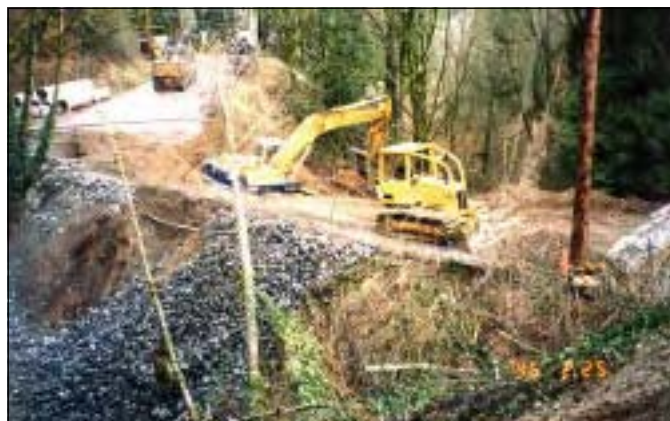
Rip rap used to provide bank stability
