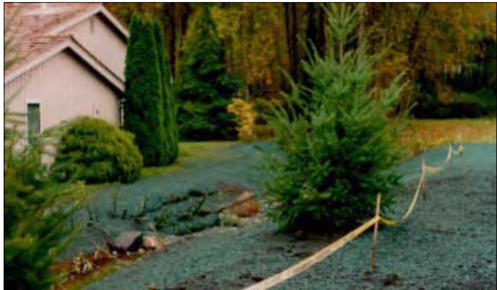
Erosion protection and vegetation establishment after maintenance work
