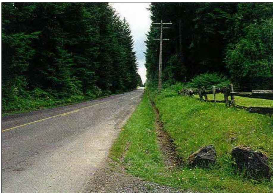
Roadside ditch with a vegetative buffer
