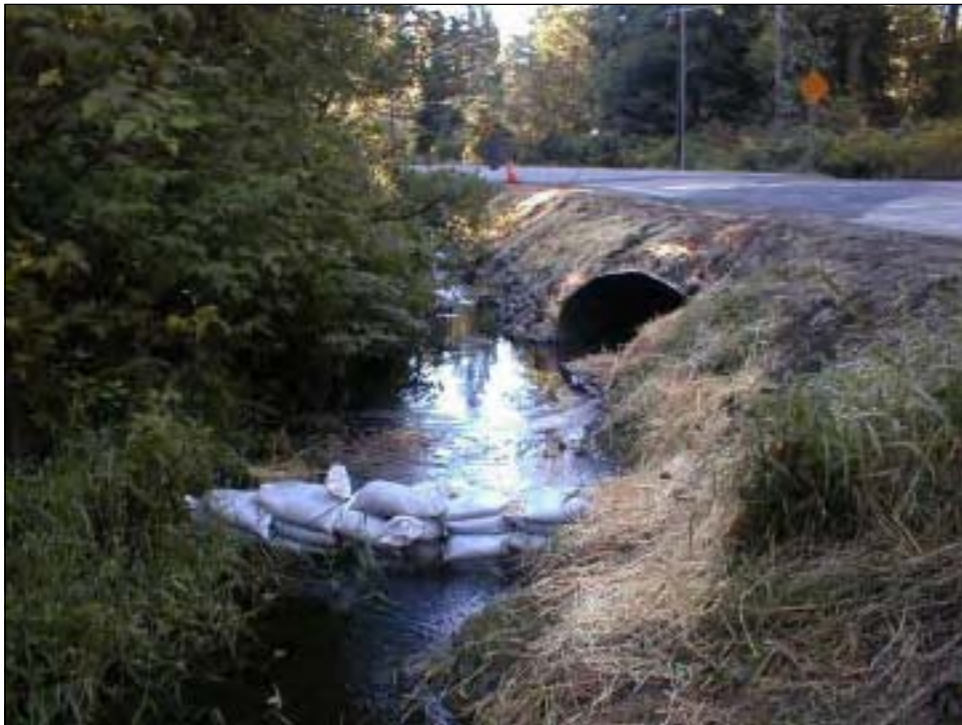
Sandbags used as a cofferdam
