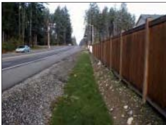
Grass lined channel: providing a filter
