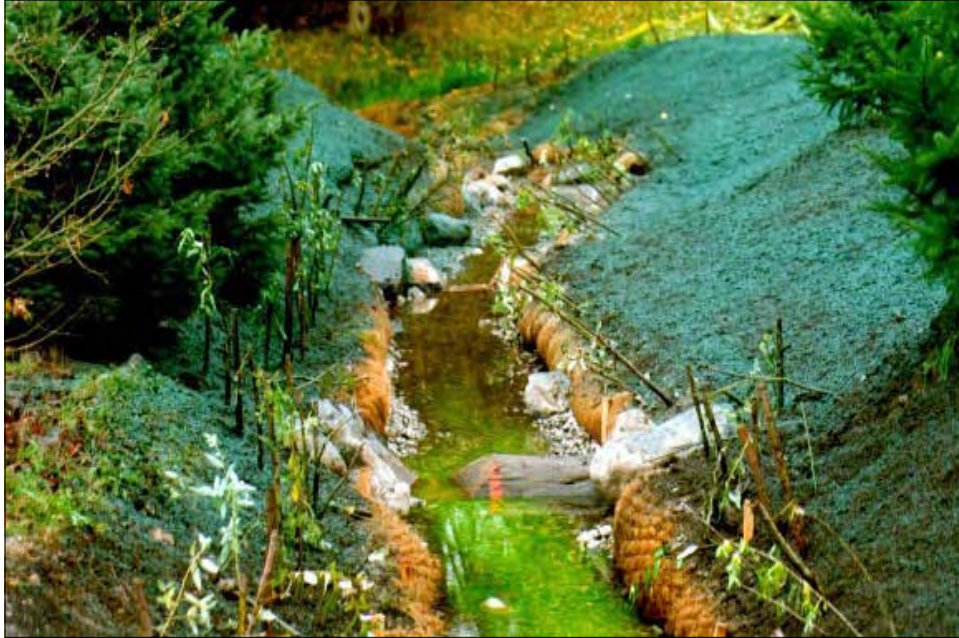
Coir logs used as habitat protection at the toe of a bank
