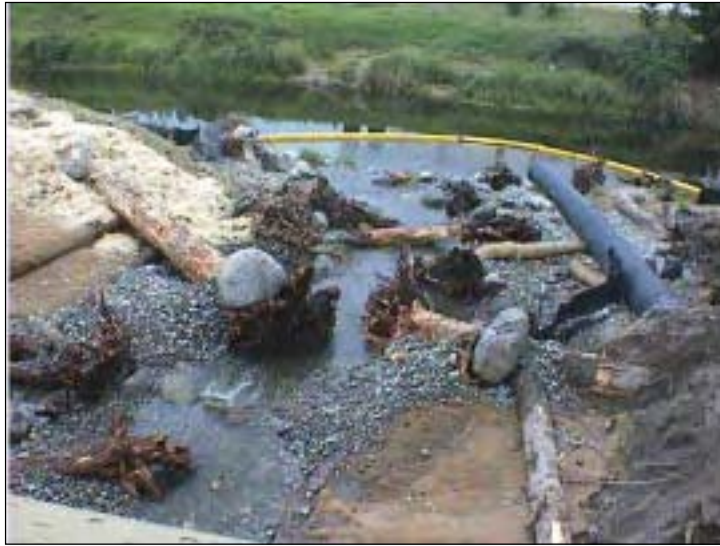
Large woody material placed in a streambed to provide salmonid refuge. Note use of turbidity curtain, streambed gravel, silt fence, coir fabric, mulching, and stream bypass
