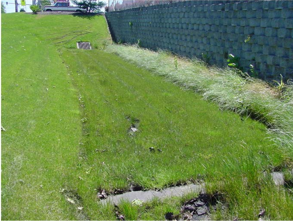
Biofiltration Swale With Spreader Bar on SR 503 in Clark County.
