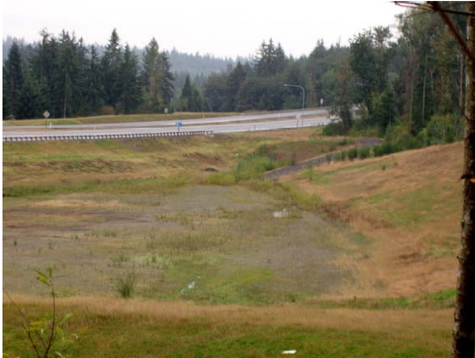
Detention Pond Along SR 18 in King County.
