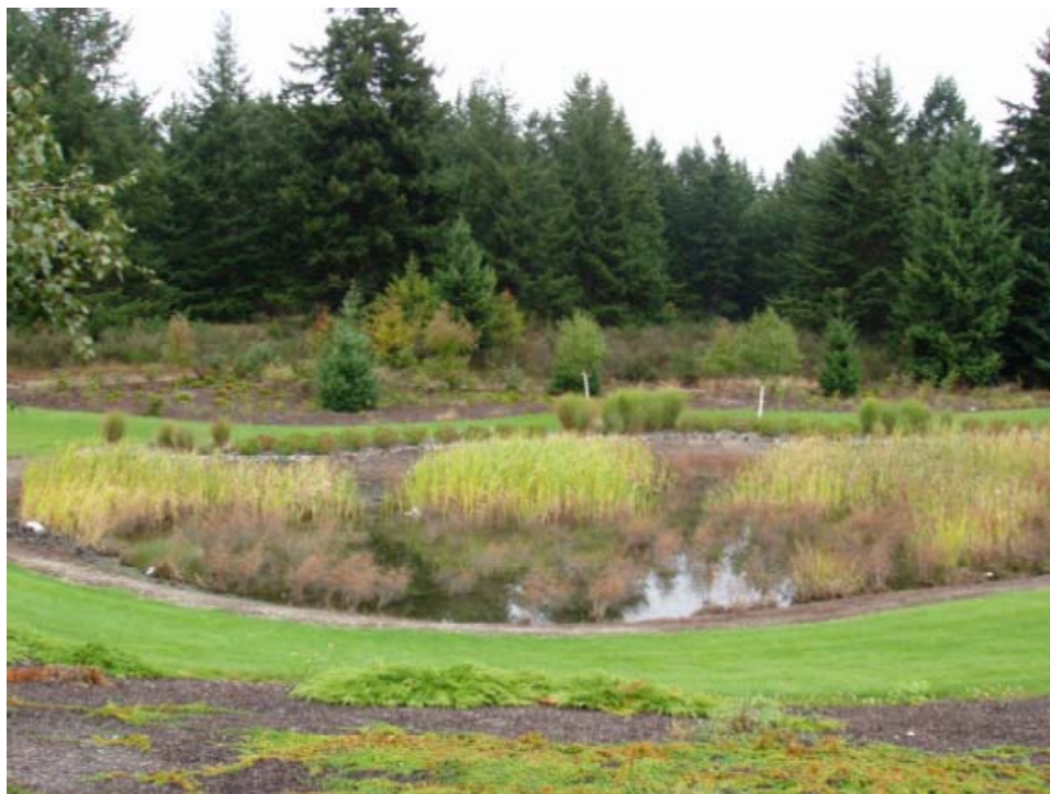
Infiltration Pond Along SR 510 in Thurston County.
