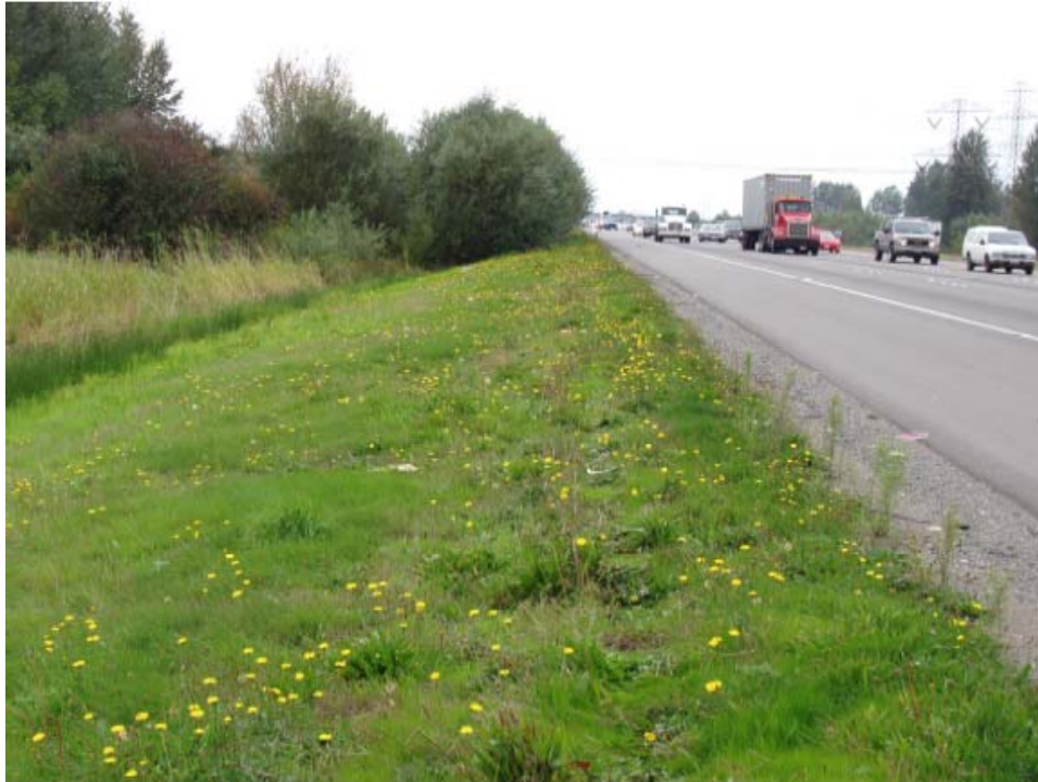
Media Filter Drain Along SR 167 in King County.
