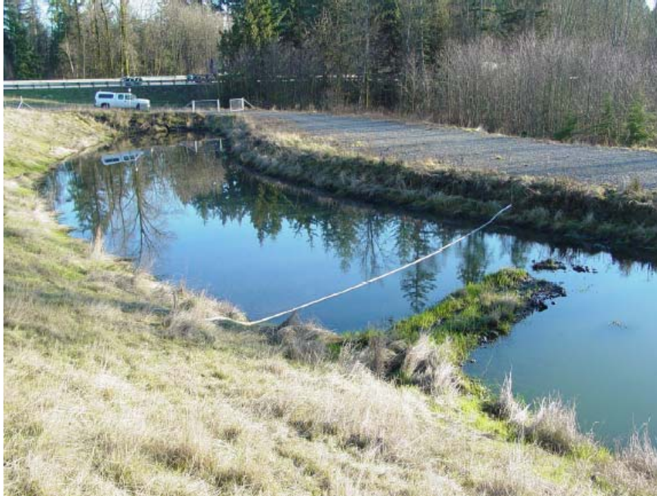
Oil Containment Boom Along I-5 in Thurston County.
