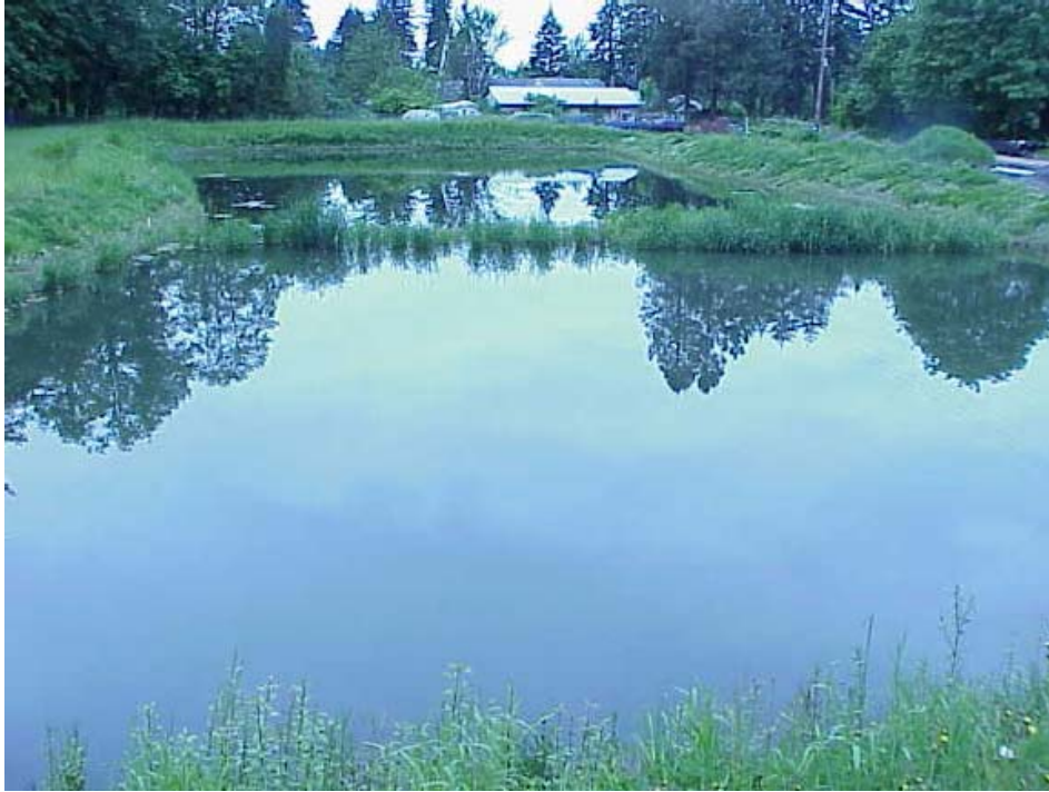
Dual-Celled Wet Pond Along I-5 in Clark County.
