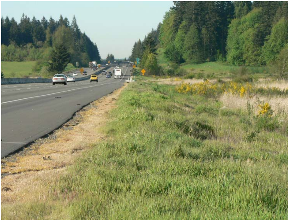
Engineered Dispersion Area Along I-5.
