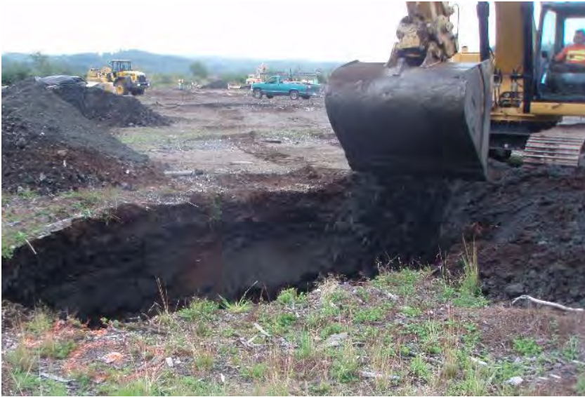
Figure 2-10. Example of Excavations Performed with a Large-Capacity Bucket without Teeth
