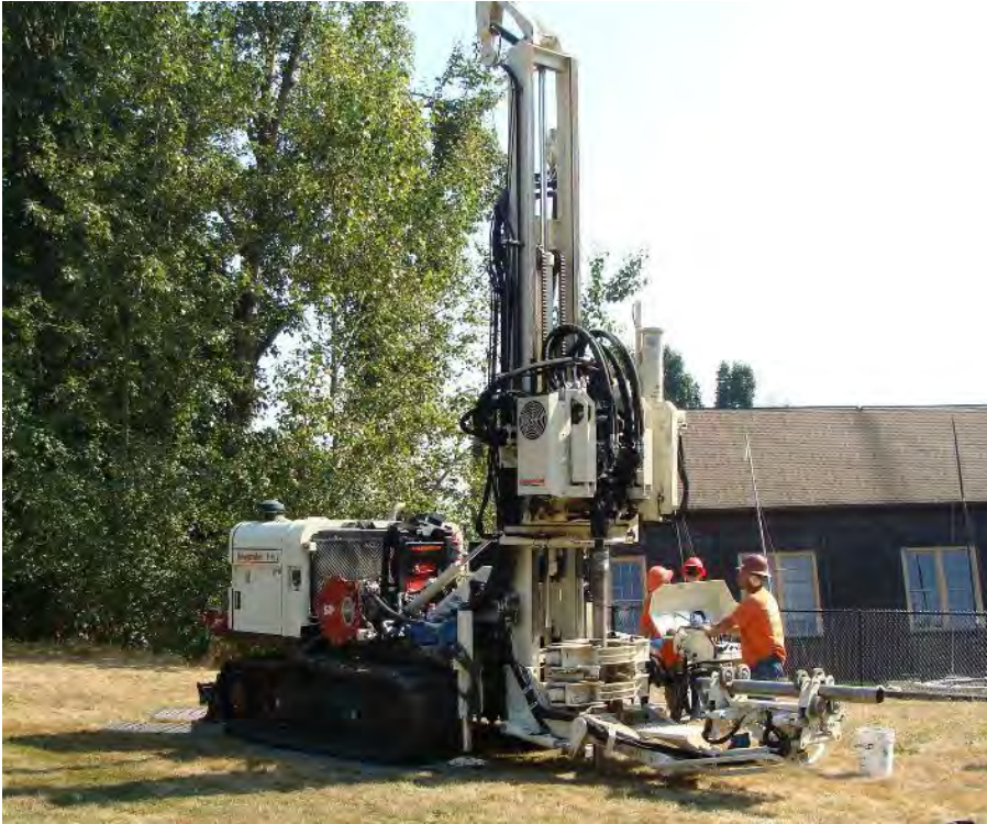
Figure 2-1. Example of a Medium-Sized Track-Mounted Rotosonic Rig with a Fully Extended Boom. The model in the photograph is a Geoprobe 8140 LS.
