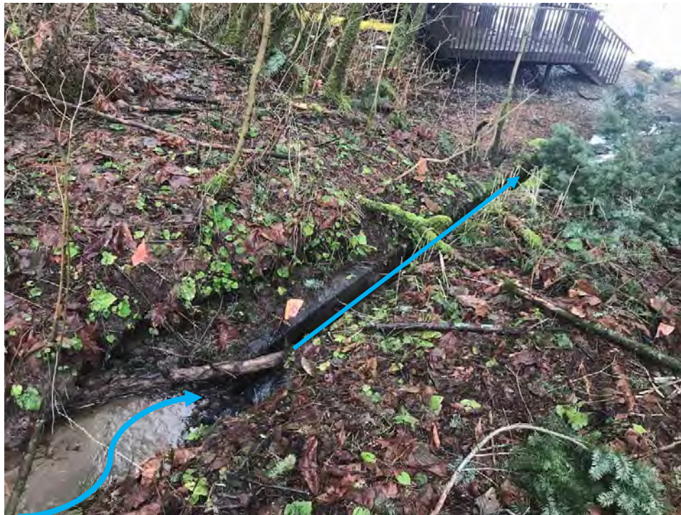
Figure 9. Concrete Structure at Stream 42, Facing Northwest
