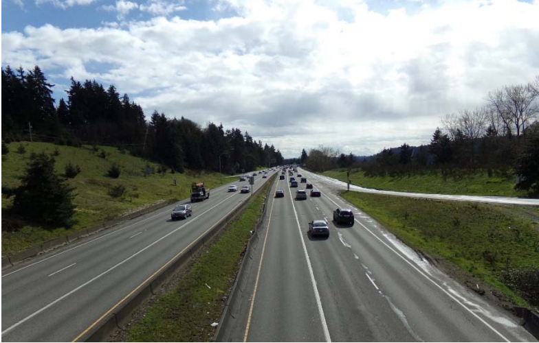
Exhibit 5-14. View G, 112th Avenue SE Interchange (Looking South) Existing Conditions
