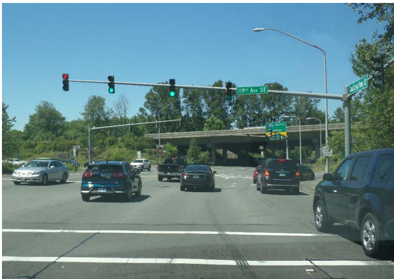
Exhibit 5-19. View J, Coal Creek Parkway Existing Conditions
