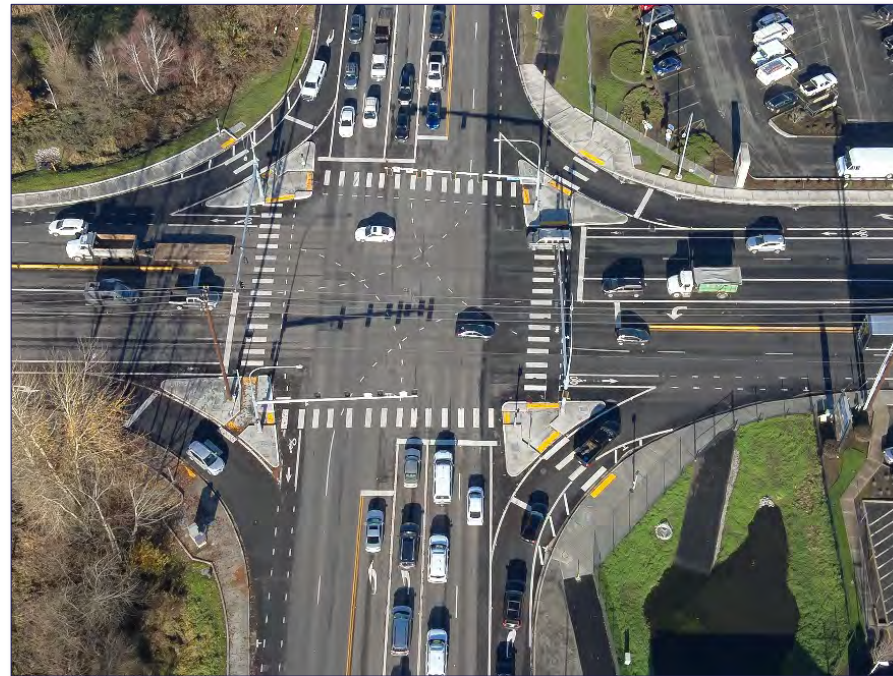
SR 502 and SR 503 Intersection
